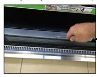
**Step 1:** Remove filter every week from lower section behind the air curtain grill.
