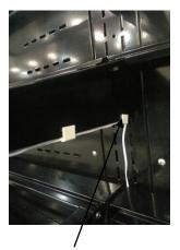
Run wire along the shelf bracket and mount using two of the supplied clips.
