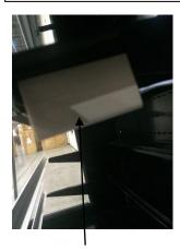
Place sensor below the third shelf from the bottom. Sensor will mount on the center left shelf bracket and positioned all the way to the front.
