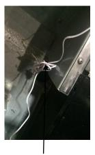
Tie off excess wire using the twist tie supplied.
